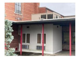
The portico is the porch between the sanctuary and the choir room, but the roof extends over the church offices which go all the way to the catwalk. This section of roof will need to be taken off and replaced. In addition, the HVAC system that sits on top of that same roof is around 20 years old. This system provides air conditioning for the sanctuary. It frequently failed last summer.
